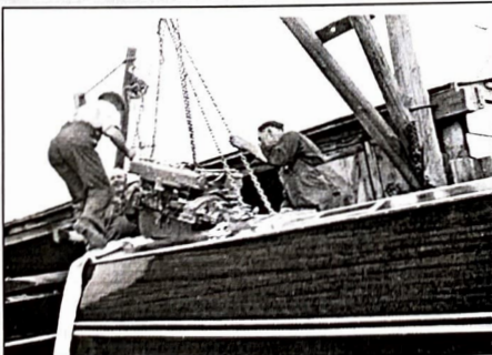
Bob and Robert Yandt installing 1939 Chrysler Crown M2 in 1940 with owner Glen Powell looking on. Photo-Yandt files
