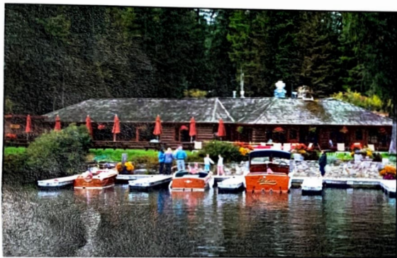
Elkins Resort 2015 Dry Rot (photo by Wes Yandt)
